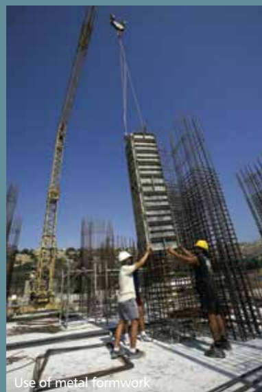
Use of metal formwork
