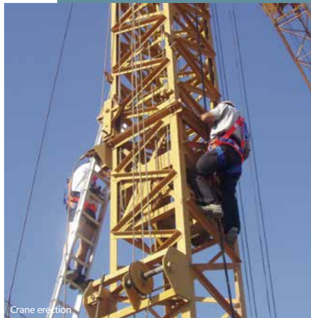
Crane erection
