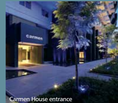
Carmen House entrance
